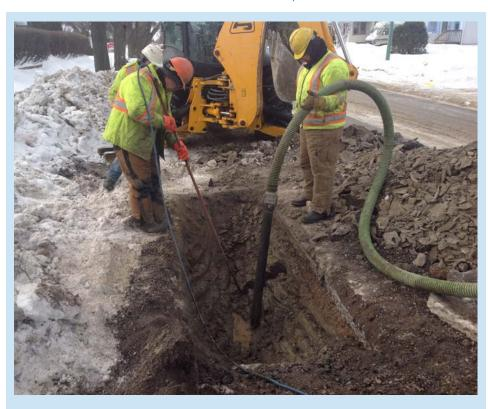
A SaskTel Crew works to install replacement cable by using hydrovac technology to run the cable underneath the roadway with minimal disruption to the street above.
